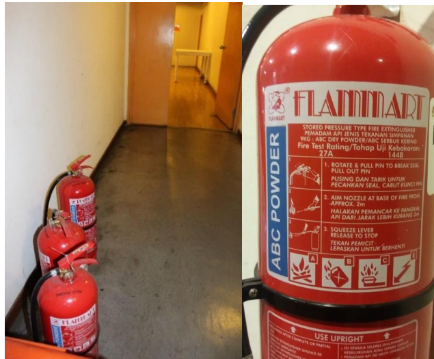
Figure 5.46: Fire extinguishers found along the emergency exit routes and along the doorways.
