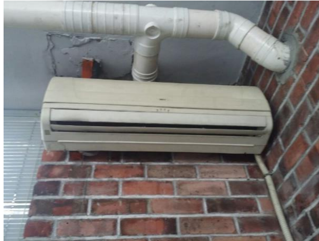
Figure 4.23: Indoor unit mounted on wall at box office Source: Sylva , (2016)
