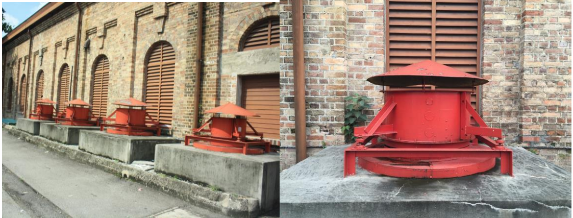
Figure 3.22 Fire exhaust fan located outside of KLPAC
