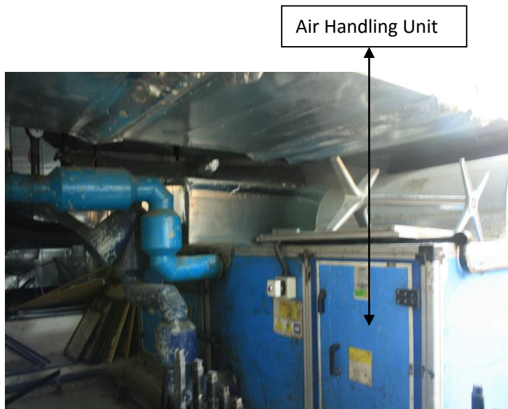
Figure 4.31: 1 of the 5 AHU rooms serving the auditoriums.
