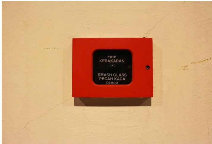
Figure 5.17: Manual call point that can be found at most of the areas and doorways.
