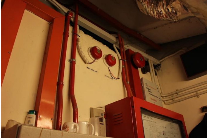
Figure 5.14: Fire alarm bells located inside the security room at ground floor.
