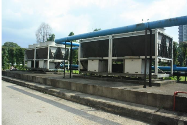
Figure 4.26: 2 air-cooled chillers used by KLPAC located beside plant room.
