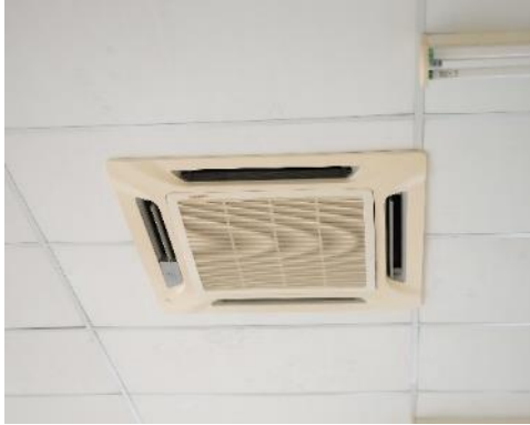
Figure 4.41: Fan coil unit at studio.
