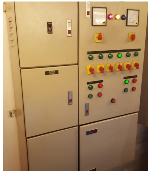
Figure 4.32: Control panel for AHU in the security room.
