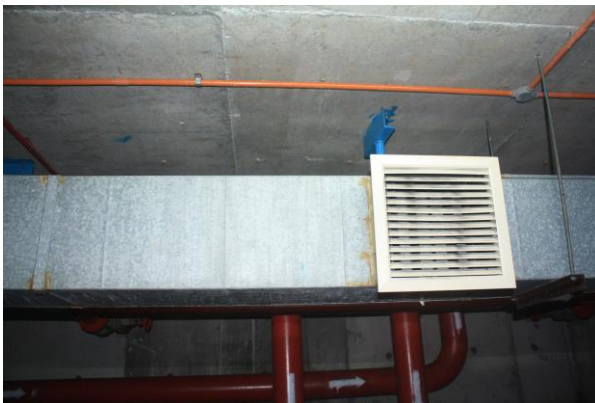
Figure 3.15: Exhaust air grille at fire pump room
