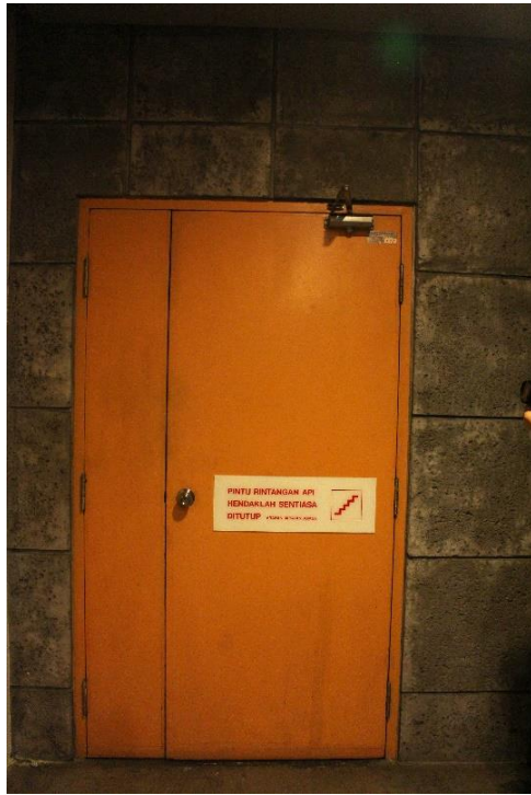
Figure 5.70: Fire rated door located at the ground floor.
