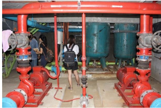
Figure 5.35: Image showing the duty pump and standby pump used for fire emergency.
