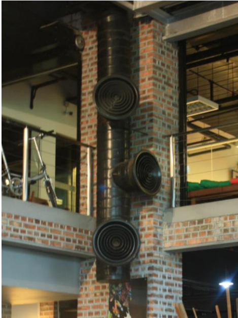
Figure 3.5: Vertical Supply Air Diffuser located in the Main Foyer of KLPAC
