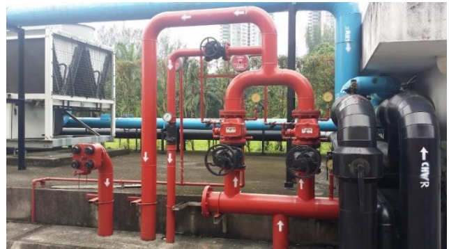
Figure 5.26: Wet pipe sprinkler system located outside of KLPAC, beside the water pump room.
