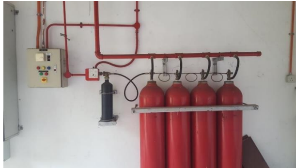
Figure 5.41: CO 2 fire suppression found in KLPAC.
