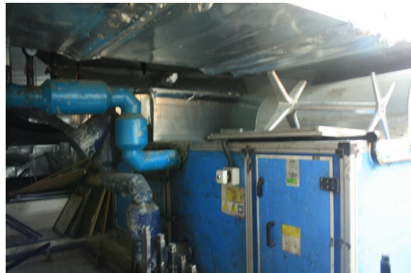
Figure 4.38: The blue casing is the sound attenuator of AHU system in KLPAC.
