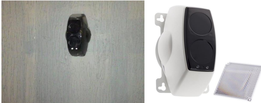
Figure 5.7: Optical smoke beam detector located at third floor and the example of the detector.
