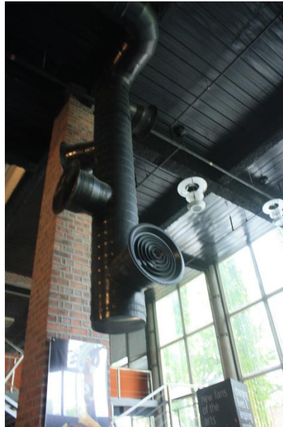
Figure4.43: Duct-like FCU in the lobby
