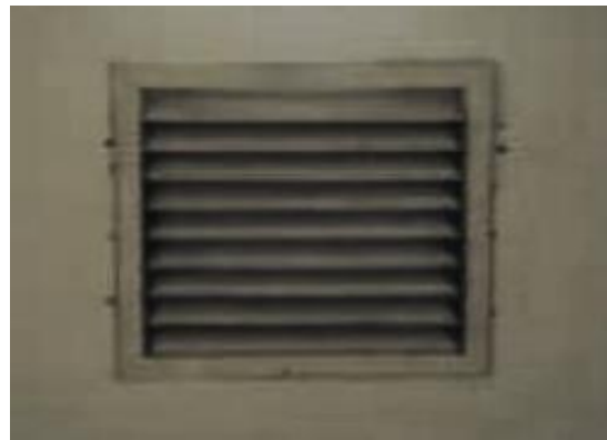
Figure 3.14: Exhaust Air Grille located on the ceiling in the toilet
