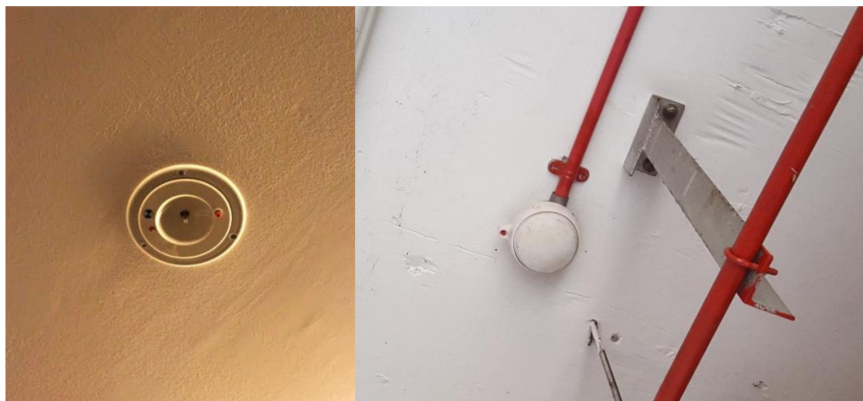
Figure 5.2: Heat detectors that are found in pre-function foyer (left) and LV main (right) at the ground floor.
