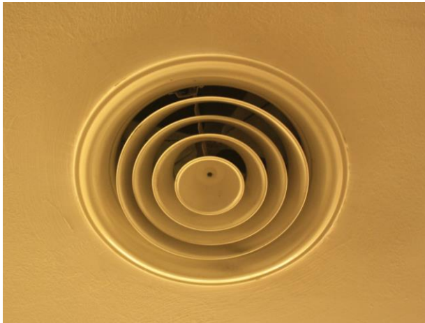
Figure 3.8 Diffuser concealed by the ceiling
