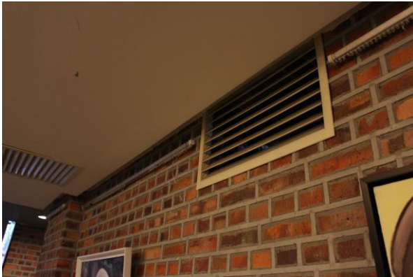
Figure 3.13: Exhaust Air Grille located at Ground Floor Corridor
