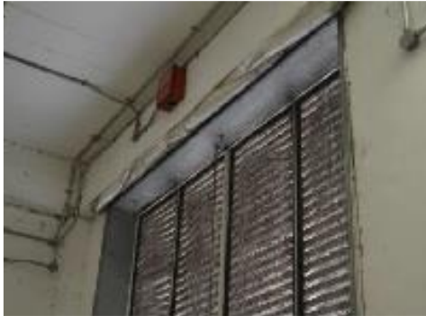
Figure 5.51: Smoke curtain found in Gen Set Room
