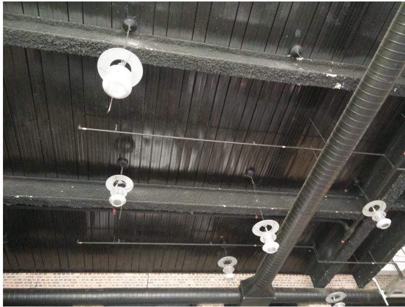
Figure 5.69: Fire proofing layer on beam.
