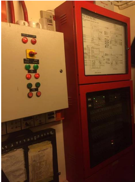
Figure 5.10: Fire Alarm Control Panel (FACP) located in the security room at ground floor.
