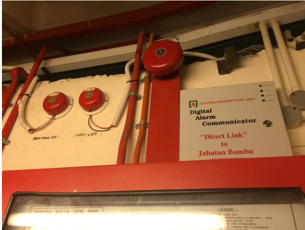
Figure 5.13: The Digital Alarm Communicator located above the control panel in the security room at ground floor.
