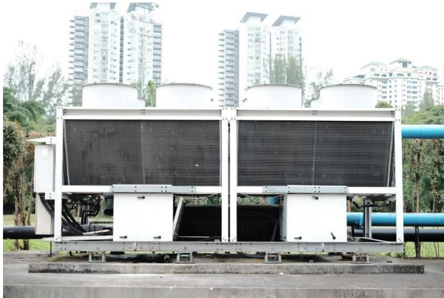
Figure 4.30: Air-cooled chiller of KLPAC.
