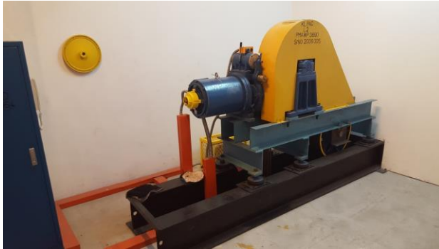
Figure 6.17 Geared Machine in KLPAC
