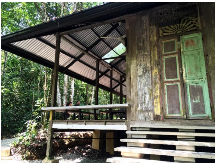
Figure 3.7 (above), 3.8 (bottom): Diagrams showing the Warehouse and Timber Shed in Sekeping Serendah that are built on stilts.
