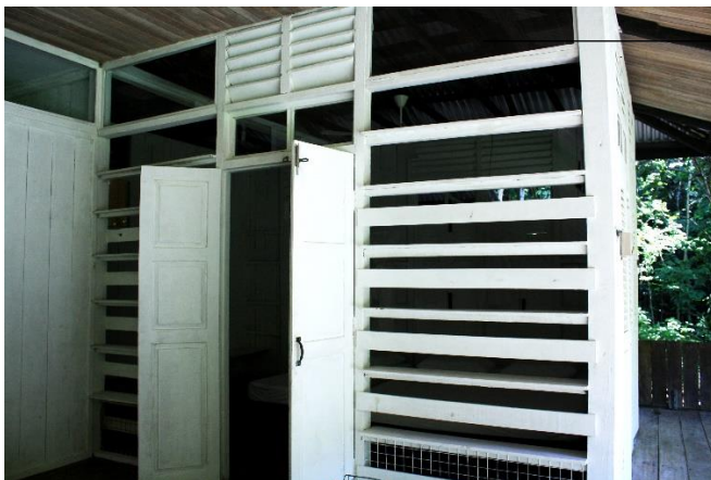
Louvre windows for ventilation purpose.
